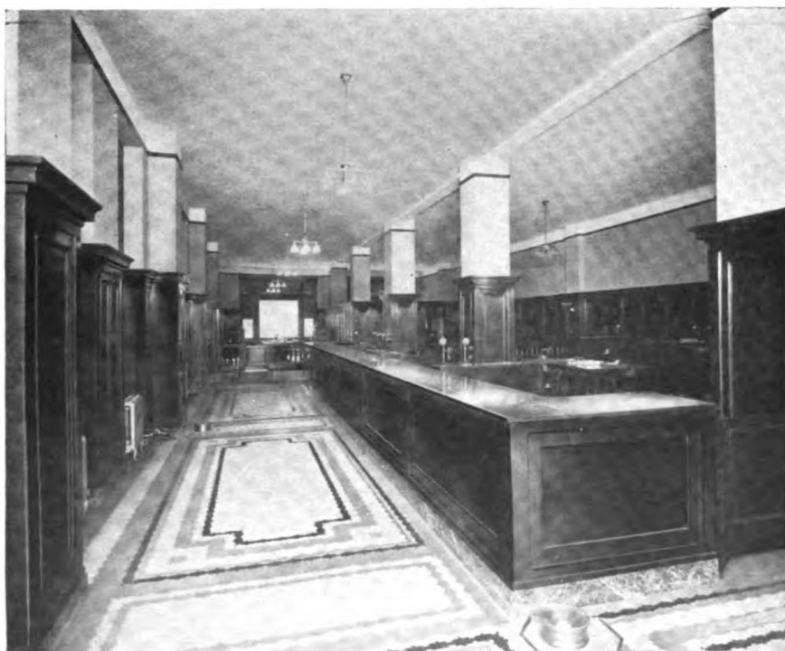
INTERLOCKING RUBBER TILING AS LAID IN THE MAIN BANKING ROOM OF HORNBLOWER AND WEEKS' NEW YORK OFFICE
